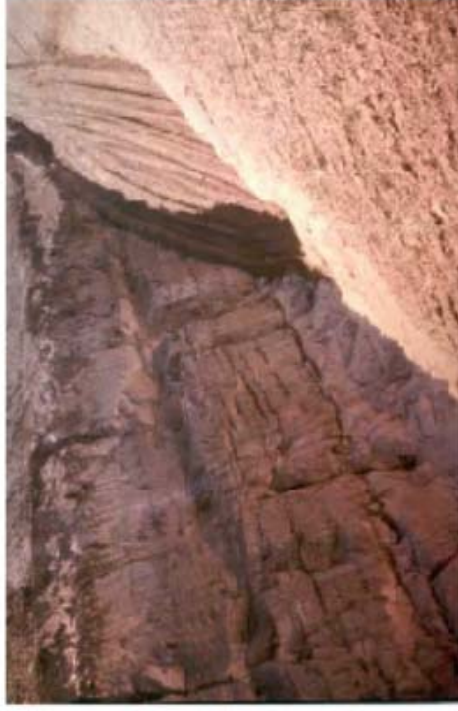
Teton Dam Core Trench and Foundation, Idaho, USA from USBR
